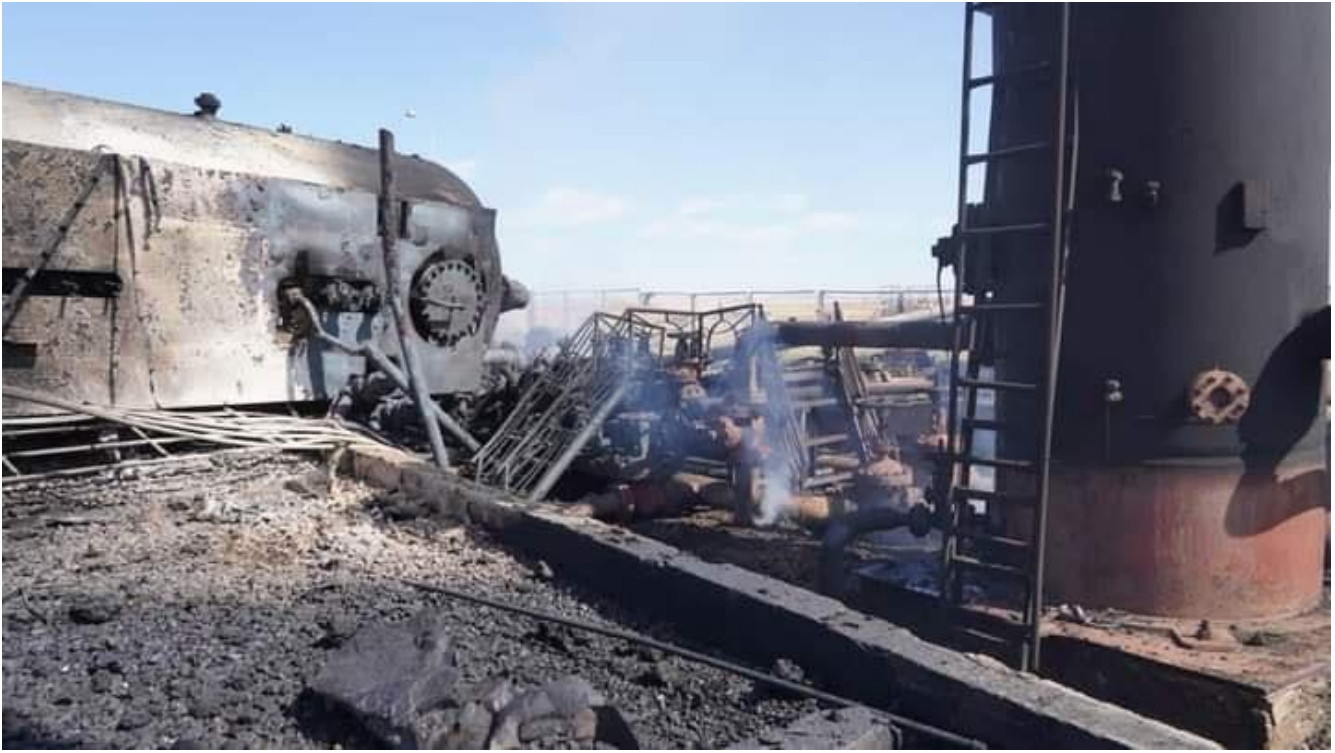
Site 3: The Sweidiya gas facility, the only gas plant in northeast Syria was put out of service by Turkish drone strikes
